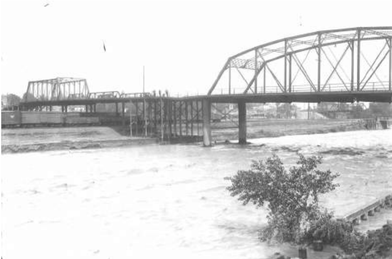
Figure 5.1. First Street Bridge over Fountain Creek at flood stage, circa 1910-12. Note the flooding at the lower right, what would have been the Lower East Side neighborhood. Pueblo's catastrophic 1921 flood destroyed the span. It was never rebuilt. (Floyd photograph, Mike Castellucci collection)
