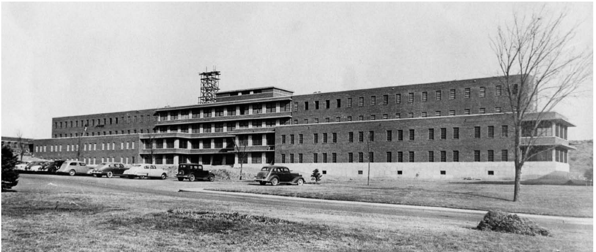
Figure 2.3. This image of the Female Building at the Colorado State Hospital was taken December 26, 1950. The four-story, brick, modest International Style building features a central bay with strong horizontal elements and recessed windows. (photo courtesy of Pueblo City-County Library District, Western History Collection)
