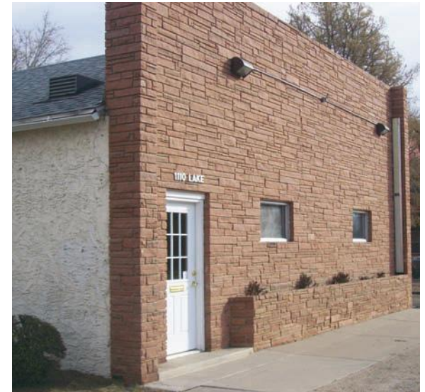
Figure 2.7. Like many neighborhood commercial buildings in Pueblo, this cottage at 1110 Lake Street had thick stone lintels over the windows before getting a postwar flagstone makeover complete with inset planter. In 1929, a grocer lived here; in 1960 it hosted Coleman Electric Company. ( Wade Broadhead )
