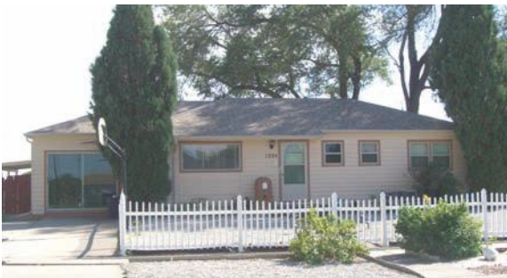
Figure 3.9. This Ranch home was John Bonforte's original construction office for the Belmont subdivision. Located at 1224 Ruppel Street, the house has been modified. Likely changes include addition of a single-car garage that was subsequently converted to living space with a sliding glass patio door on the façade. (Mary Therese Anstey)
